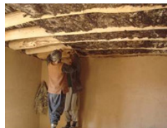
Figure 1.17: internal roof thermal insulation
