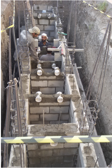
Figure 4.7: Settler, ABR and AF during construction
