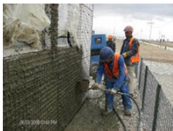
Figure 1.15: External wall thermal insulation
