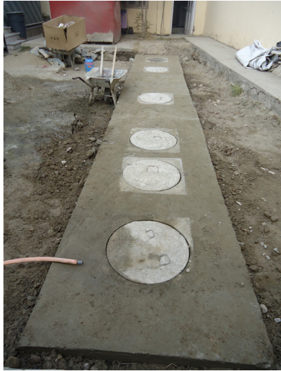
Figure 4.8: Settler, ABR and AF After construction
