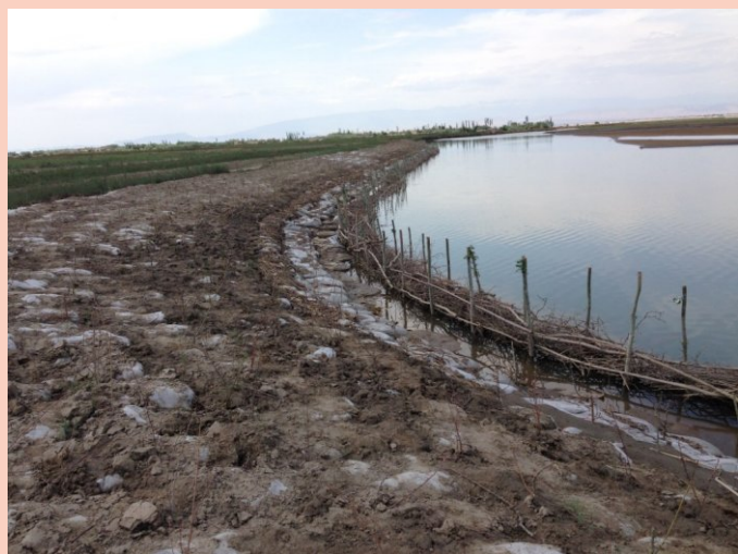
Amu River Bank; Before, During and After construction of bio dykes.
