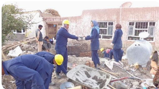
Women working at Biogas building Site
