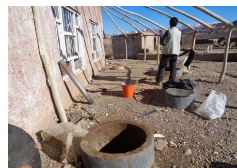
Picture.2 Toilet Linked Biogas Plant in Bamyan (Courtesy of BORDA Afghanistan)
