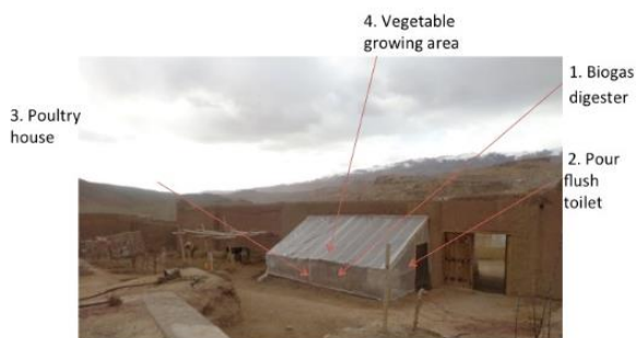
Figure 1. Biogas 4 in 1 system, Bamyan district, Afghanistan.
