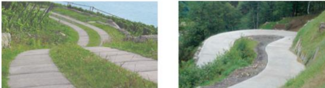
Photo 1: Sample of proposed concrete pavement – concrete pavement in curves – steep road sections and track lane at steep road sections
