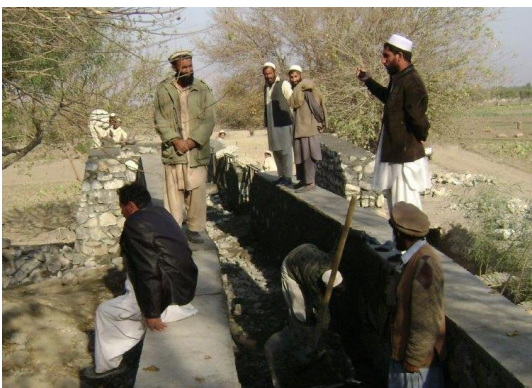
Canal-lining project Nangarhar province, National Solidarity Program. Photo: The IRC
